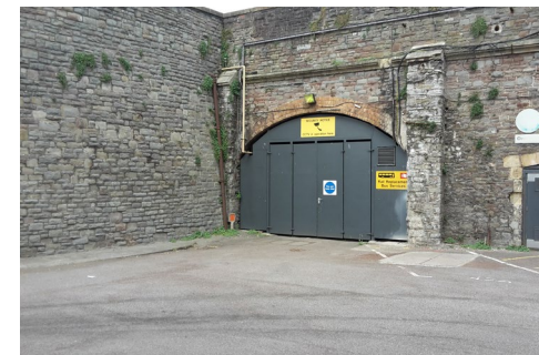
Figure 122 Bristol & Exeter Yard rail replacement area
